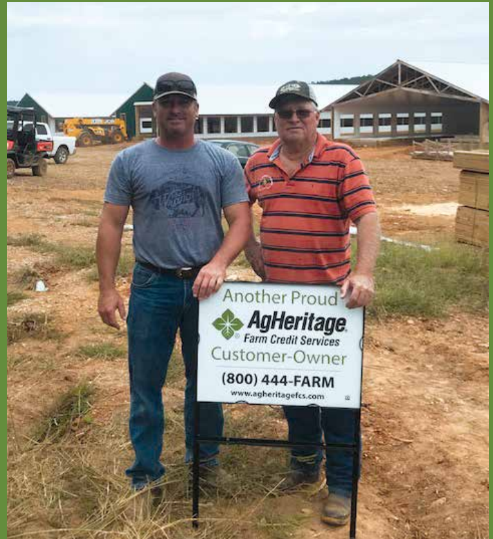
Pocahontas Branch customer-owners Joe Reel and son Brian Reel launch their new poultry operation with Peco Foods, Inc. by building four new breeder houses.
